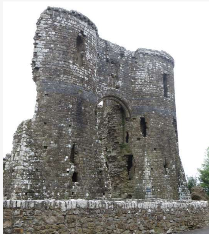
Curtain walls, here the gate towers of Llawhaden Castle, Wales © the Author.
